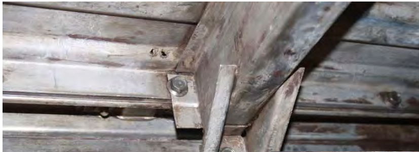
Removing and cleaning the body bolts separately helped.
